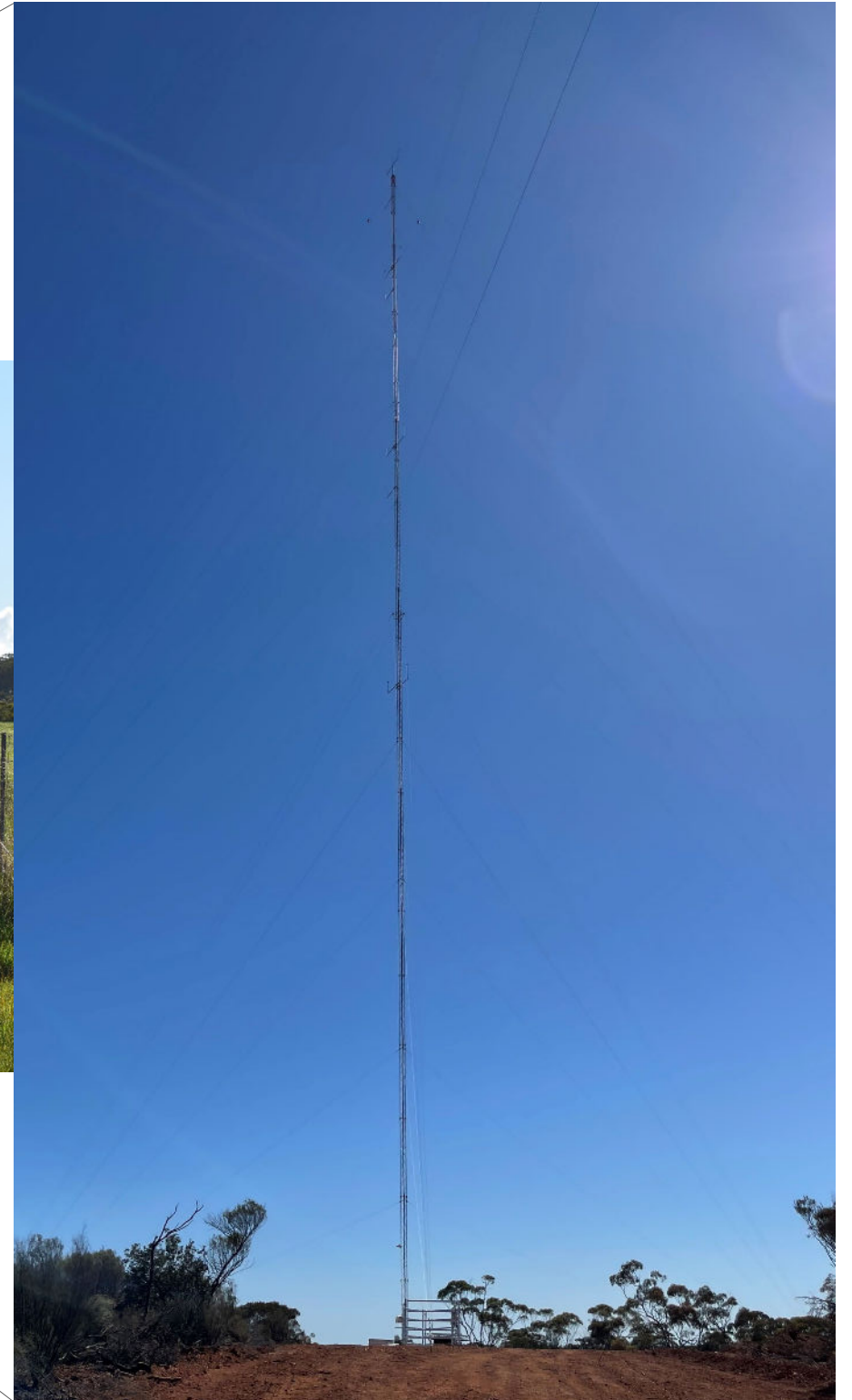
Indicative Meteorological Mast arrangement (close up view)
